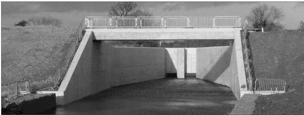
Figure 3. Huscote flow control structure, looking upstream
