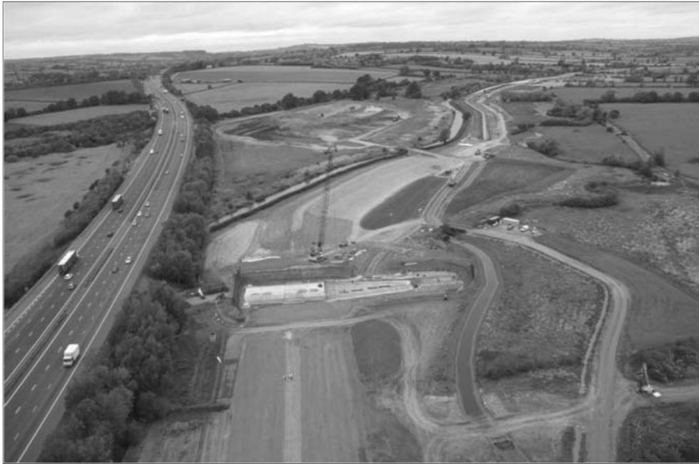
Figure 10. Embankment, Hardwick control structure and borrow pit (09/11)
